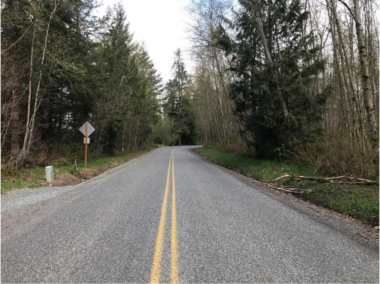
Gripp Road near entrance /exit to Haul Road
